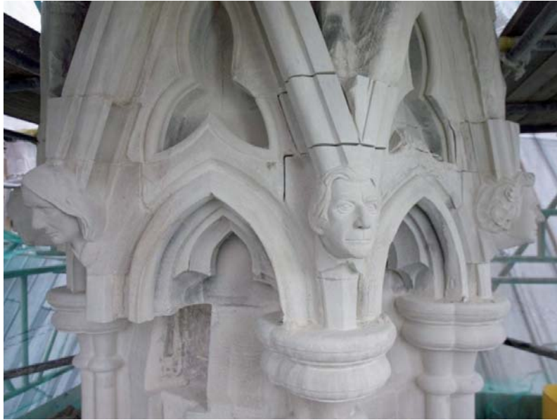
Pinnacle - work in progress
