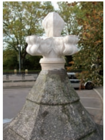
A finished finial in position at London City Cemetery (Photo: Katie Worthington, by courtesy of Stonewest Ltd)
