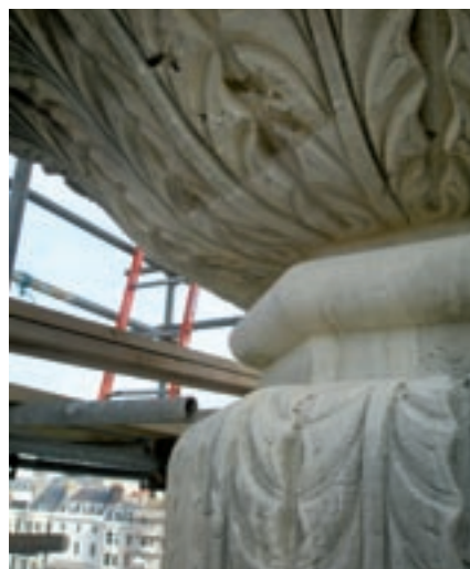
Detail of the new carving and its back after being 'keyed up' with an angle grinder (Photos: Katie Worthington, by courtesy of Stonewest Ltd)
