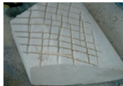
Detail of the new carving and its back after being 'keyed up' with an angle grinder (Photos: Katie Worthington, by courtesy of Stonewest Ltd)
