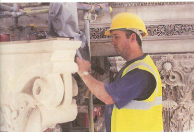
Stonewest carver Dave Baker carving a one tonne piece of Portland stone that has replaced the top part of a Corinthian capital on a pillar on the south-east elevation.
