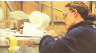
Kate Worthington from Stonewest carving some of the replacement stonework in a mason's shop set up on site.
