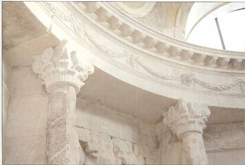
Above. In the chapel, damaged capitals and mouldings have been repaired and, where necessary, replaced. The plaster dome (pictured below) has also been repaired by PAYE. A white marble reredos and Brocatello cladding to the columns are now being installed in phase two of the project.
