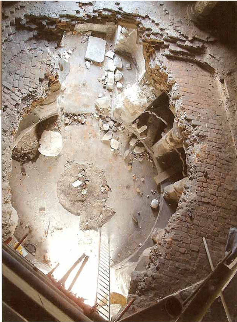
The vaulted Portland stone over brick roof of the crypt supporting the stone floor of the chapel above had collapsed (above) in the face of extreme attacks. PAYE restored the roof, the floor above it and the severely damaged plasterwork of a dome over the chapel.
