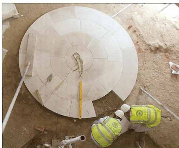
The vaulted Portland stone over brick roof of the crypt supporting the stone floor of the chapel above had collapsed (above) in the face of extreme attacks. PAYE restored the roof, the floor above it and the severely damaged plasterwork of a dome over the chapel.
