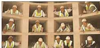
Darnley Mausoleum restoration (p26)
