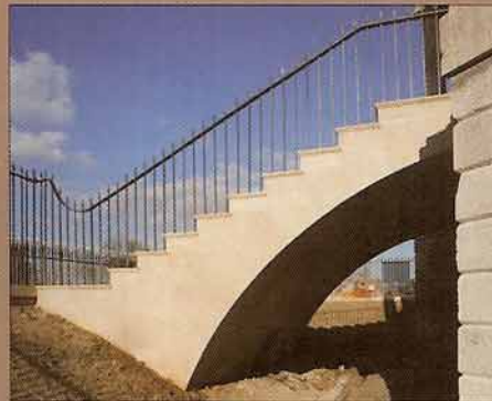
A new flying bridge in Portland limestone.
