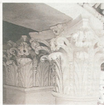
St Paul's shrouded in scaffolding, above, and, left, a restored capital carved on the south west tower
